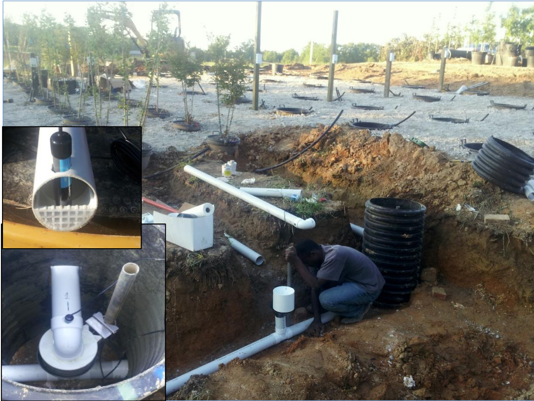
Fig. 31. Installing the sensor network control block at Hale and Hines Nursery. Here, ECRN-100 rain gauges are being integrated into the drainage line, to quantify leachate from the ten trees in each row. Inset pictures at left show in-line EC (ES2) sensor in cross-section and from the top, where the drainage line enters the rain gauge.
