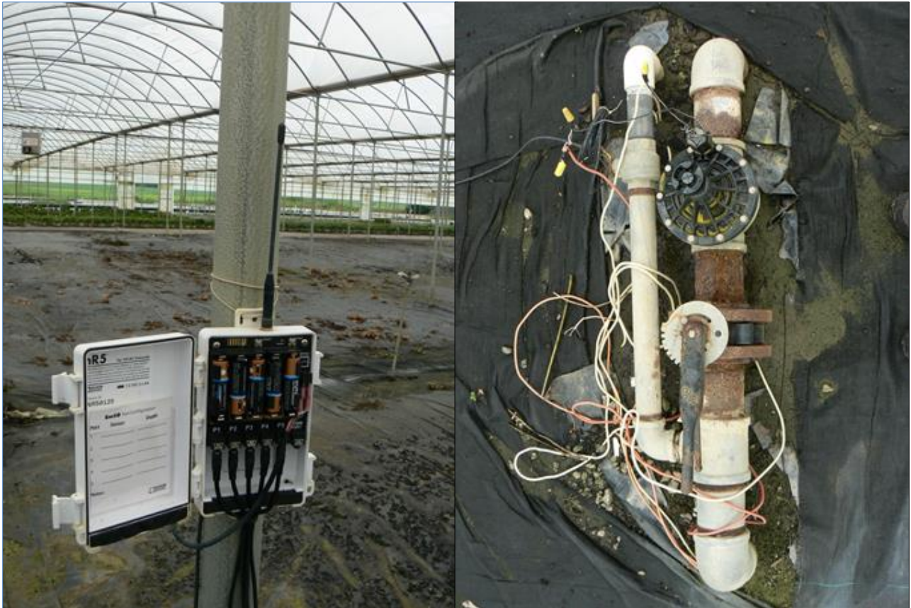
Fig. 20. An nR5 irrigation control node in the 4-acre greenhouse at McCorkle Nurseries (left) controls water flow through a 4" water line (right), using a standard 24 VAC solenoid. Note the lack of plants in the area around the irrigation control node. Irrigation decisions are made using data collected by an EM50R node that is placed in the crop in the background. Sensorweb's 'global control' allows the nR5 node to irrigate based on sensor readings from another node in the wireless sensor network.
